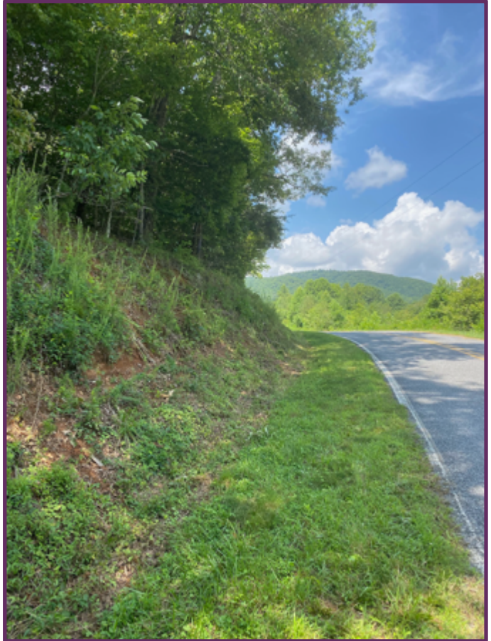
Location 3 Road Cut
