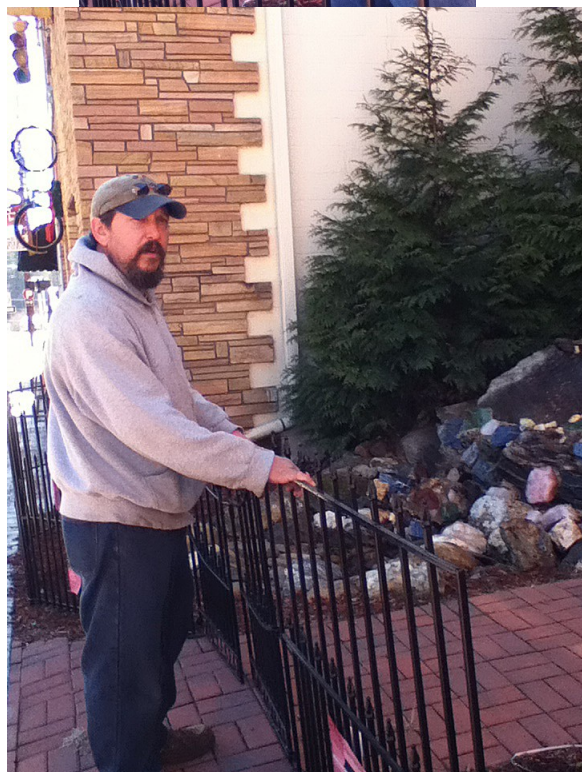
Lon Peden and Tom Sterrett pictured working on iron fencing.
