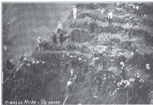
FIG. 12.—PHOTOGRAPH SHOWING "PEONS" WORKING ON A BANK, BREAKING DOWN THE EMERALD FORMATION WITH LONG, IRON CROWBARS.
